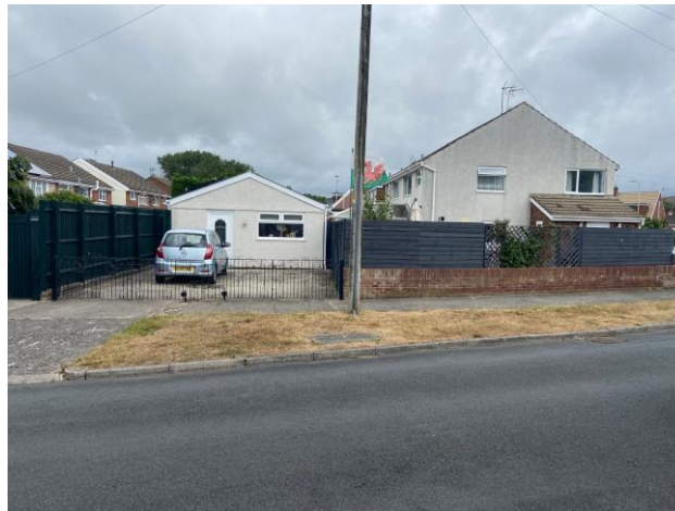
Fig. 6 - The existing driveway to be widened
